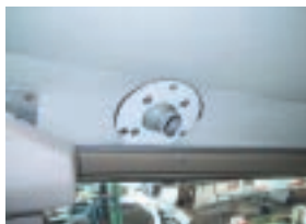
Old air ventilation valve.
